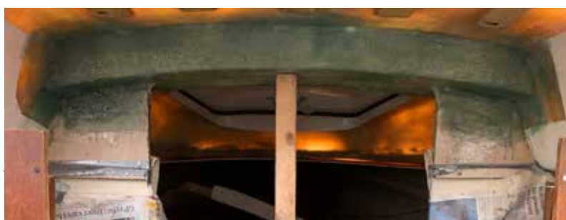
Nya balken plastas fast.
